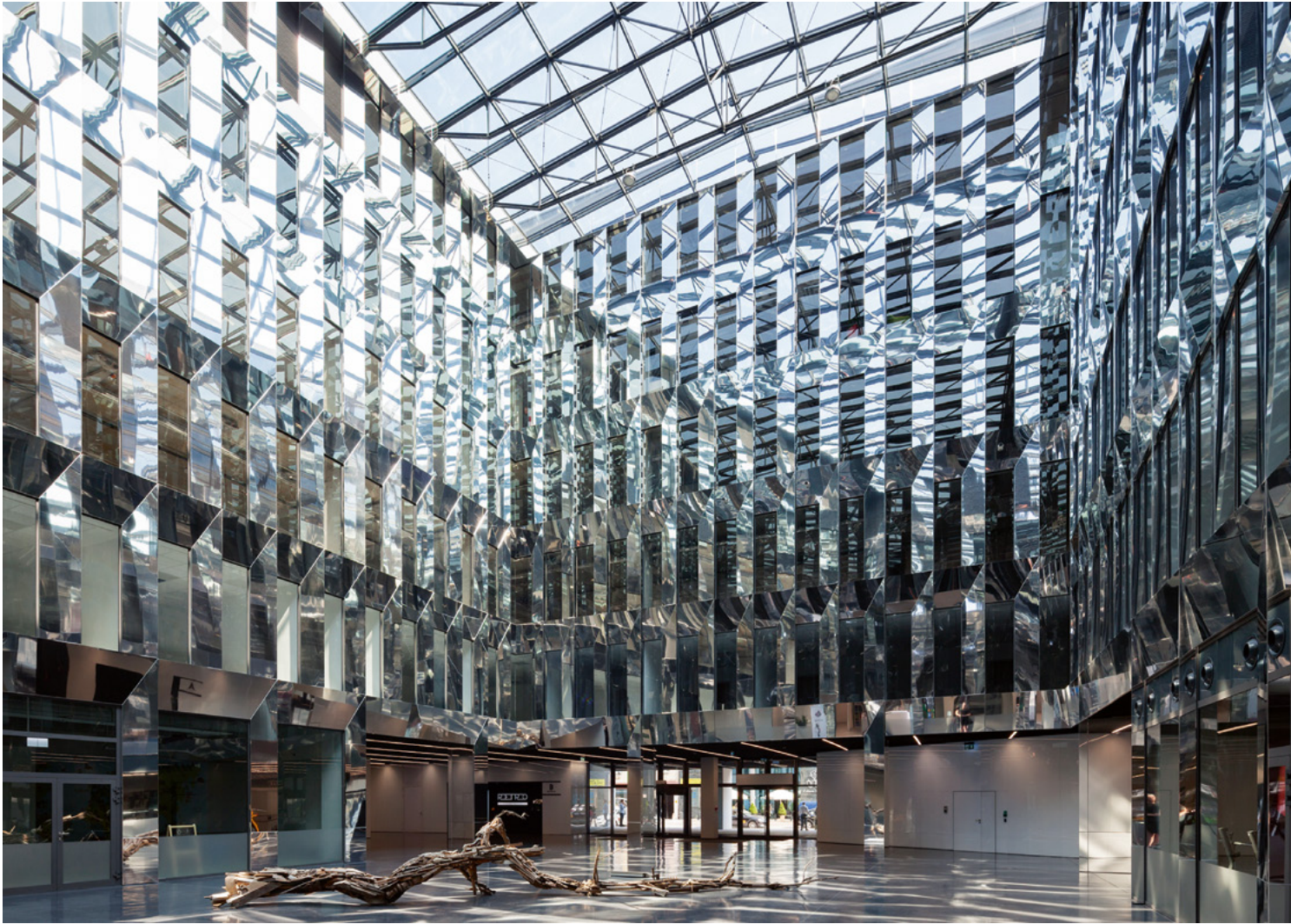
The Retro Office House in Wrocław, Poland is made with mirrored panels in DECO PRIME® 4, scattering the light from the glazed roof
