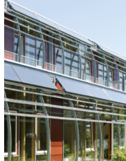
Solar thermal system with absorbers from Alanod at the Albstadt State Sports School
