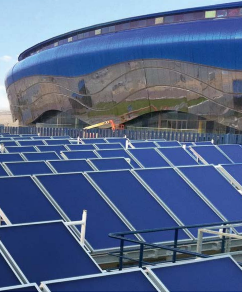
Hamdan Sports Complex, Dubai, UAE, with 1,026 m 2 flat plate collectors to heat swimming pools, under floor heating and domestic hot water
